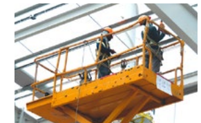
Aerial work platform at construction site
