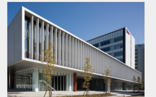
IDEC Head Office / Technology Research Center
